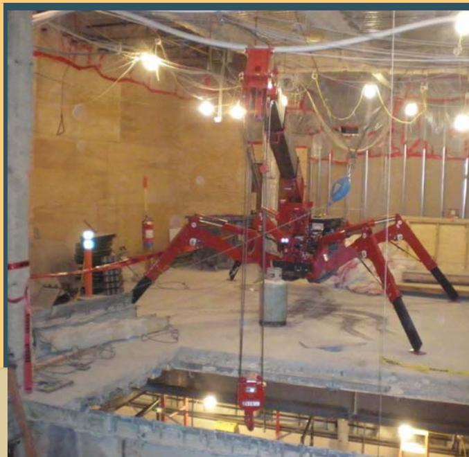
The Spider Crane is helping with steel construction on the Central Court Building Escalator Project.
