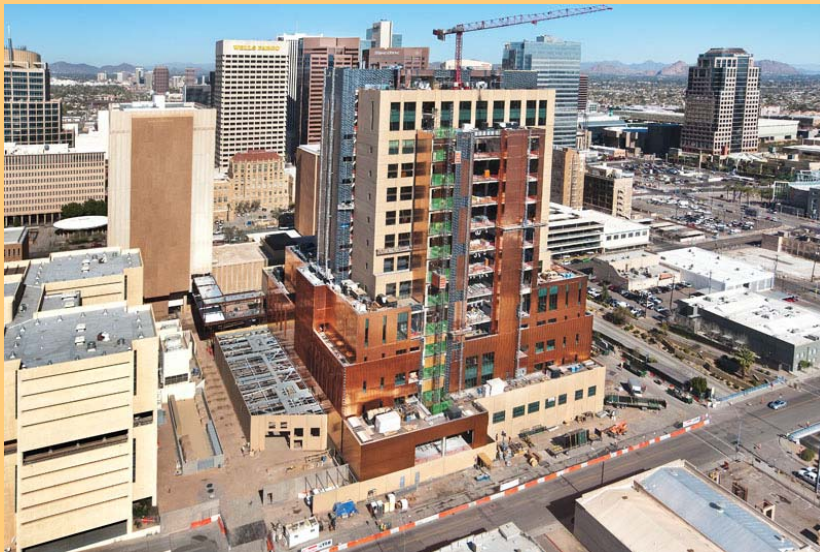
Photo by Maricopa County Court Tower Construction Update
