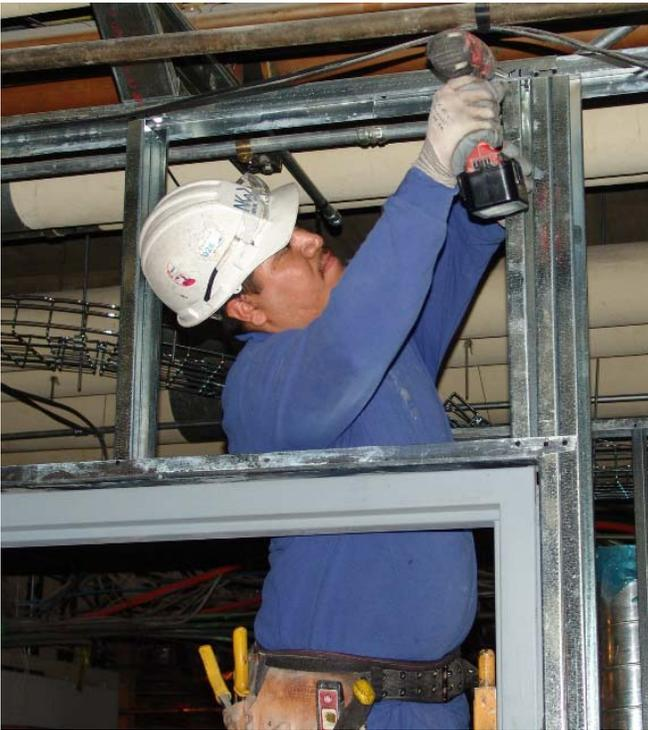
*A construction worker frames one of the new RCC courtrooms in the basement of the Central Court Building. The courtrooms are expected to open in June of 2009.*
